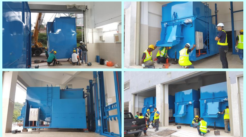
INSTALLATION OF THE SPIRAL WASTE BIN SYSTEM AT PROJECT SITE
