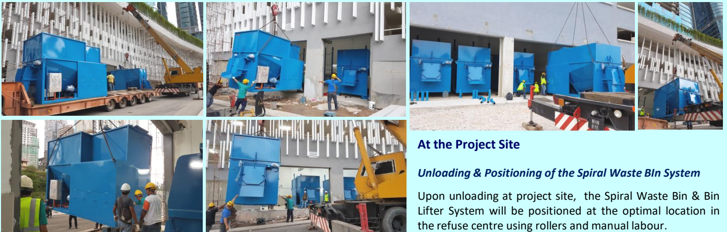
UNLOADING OF THE SPIRAL WASTE BIN SYSTEM AT PROJECT SITE
